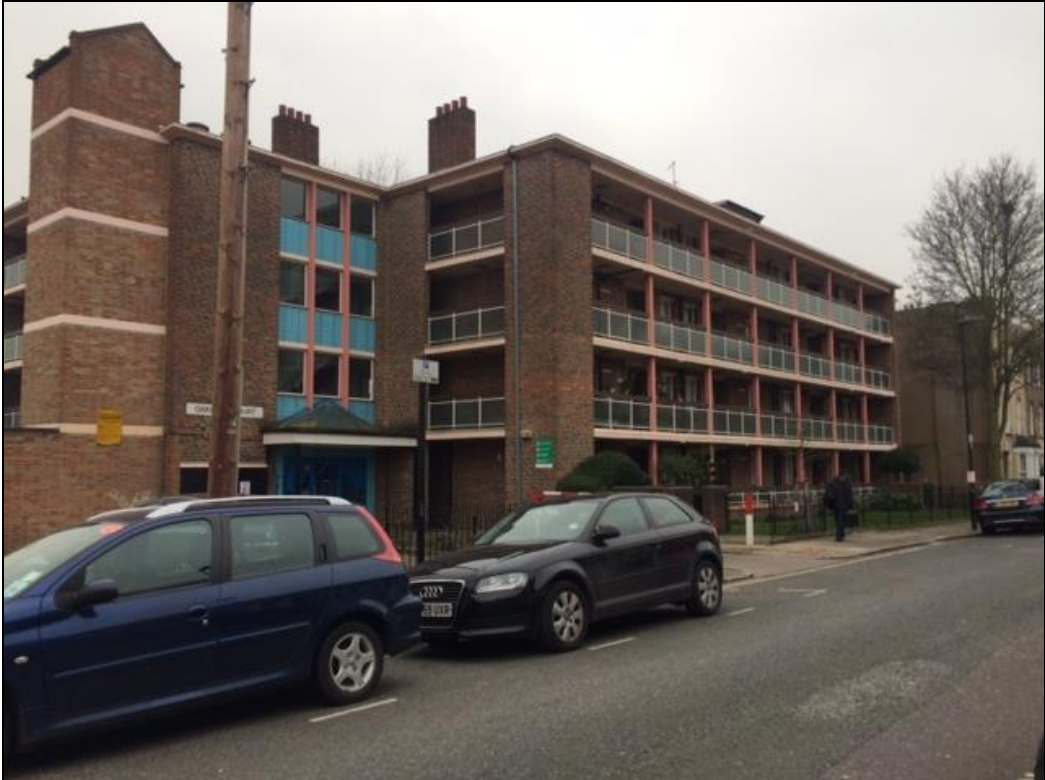
Image 1: Front Elevation of Building
