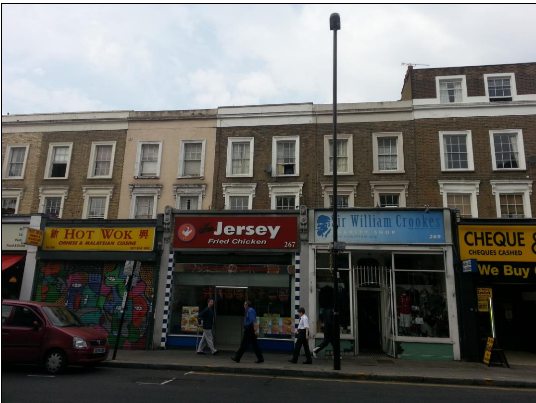
Image 1: The front of the building from Caledonian Road
